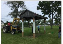
Here's how the work unfolded - once the nuts and bolts were removed to make the roof removal possible, the "Old Ford" moved in and lifted the roof from the legs. But wait, the legs had to be put on the trailer first to support the roof structure. Out came the chainsaw - watch out for those toes, I thought! The legs were cut off as close to the ground as possible and you could hardly tell that there had ever been any such structure there at all.
